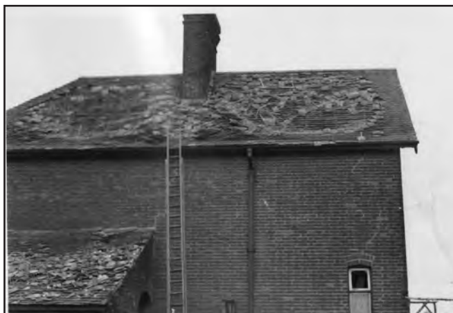
This damage was caused on 13 Oct 1944 when a buzz bomb blew up just after it passed this house in Little Fransham. A woman was injured when the roof collapsed; she was later treated by a 392nd BG doctor.
