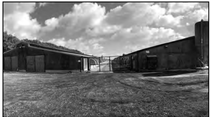
The main runway, made of concrete, was 6,000 feet long. The turkey huts show how wide it was.
