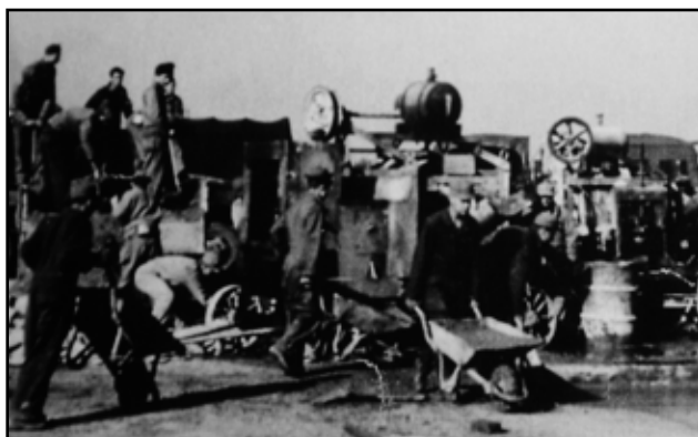
Top: When 392nd BG ground personnel arrived at Wendling, they found mud everywhere. Bottom: One early task was to pour concrete for additional hardstands and new roads throughout Station 118.
