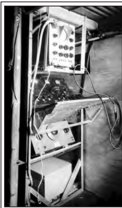
The 36th Bomb Squadron was the only unit in the 8th AF completely dedicated to Radio Counter Measures (RCM). This photo shows their S-27 radio equipment, which typically had more components than what the voice interpreters used. Photo from http://www.36rcm.com/equipment/equipment.htm
