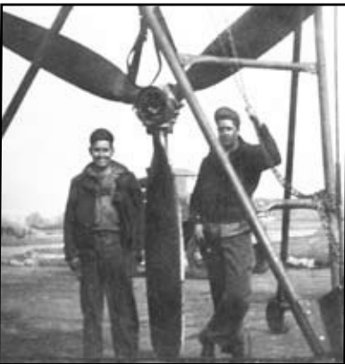
576th Sqdn ground crew personnel change an engine (top photo) and propeller (bottom photo). The a/c would then be taken for a test spin before it was returned to combat. The old engine would likely be sent to a depot for overhaul or salvage. This kind of maintenance work went on daily, outside, regardless of the weather. Both photos from 576th crew chief M/Sgt Walter S. Meeker.
