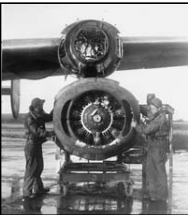
576th Sqdn ground crew personnel change an engine (top photo) and propeller (bottom photo). The a/c would then be taken for a test spin before it was returned to combat. The old engine would likely be sent to a depot for overhaul or salvage. This kind of maintenance work went on daily, outside, regardless of the weather. Both photos from 576th crew chief M/Sgt Walter S. Meeker.
