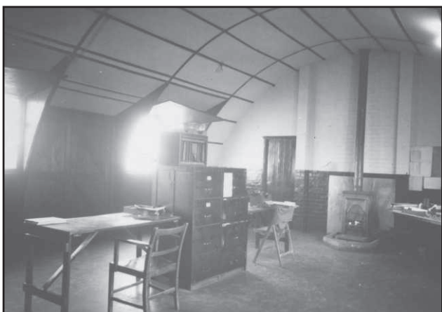
Top: LtCol Peter Nissen (left) and one of his huts in 1917. Middle: Two 392nd BG Nissen huts. Bottom: The Station Orderly Section on 20 Feb 1945. The interior framing is clearly visible, as are dormer windows, doors at the back and side, and a stove.
