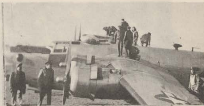
Aircraft #594 lands with collapsed gear, February 17, 1945.
