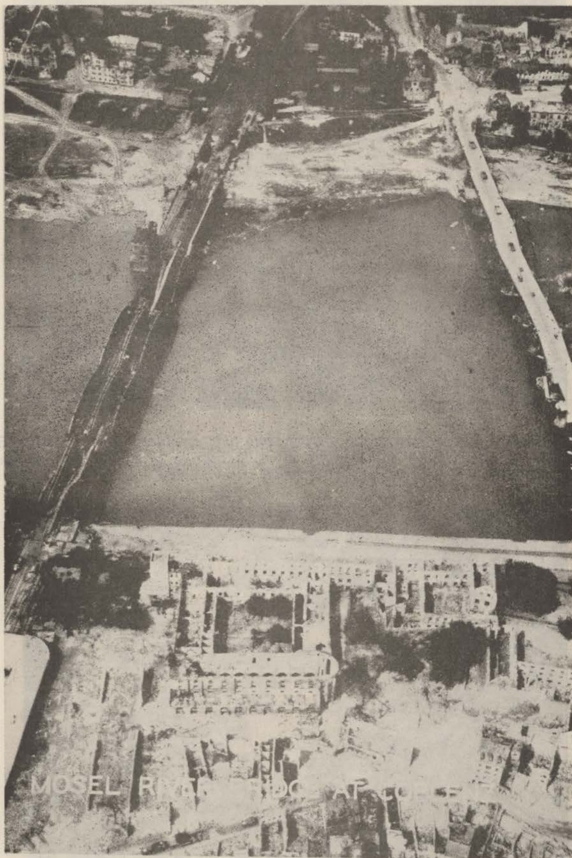
MOSEL RIVER BRIDGE AT COBLENZ
