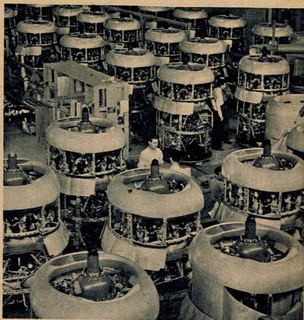
FINAL ENGINE ASSEMBLY for Liberators. Pratt & Whitney 1200 HP. engines mean power with a capital P.
