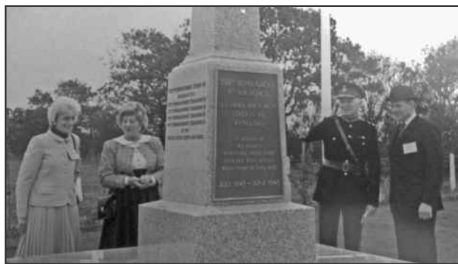
On 7 Oct 1989, Jill Scott, at far left, and Tom Scott, at far right, admire the newly renovated Memorial.
