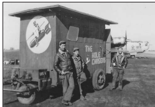
Pvt Rudy Santelli (2nd from left) and other 577th sheet metal workers with their repair shop, "The Hole Chasers." They moved it from plane to plane to patch holes caused by flak, bullets, and rockets. #42-95079, Puss 'N Boots, is in the background.
