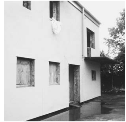
New restored control tower at Rackheath
