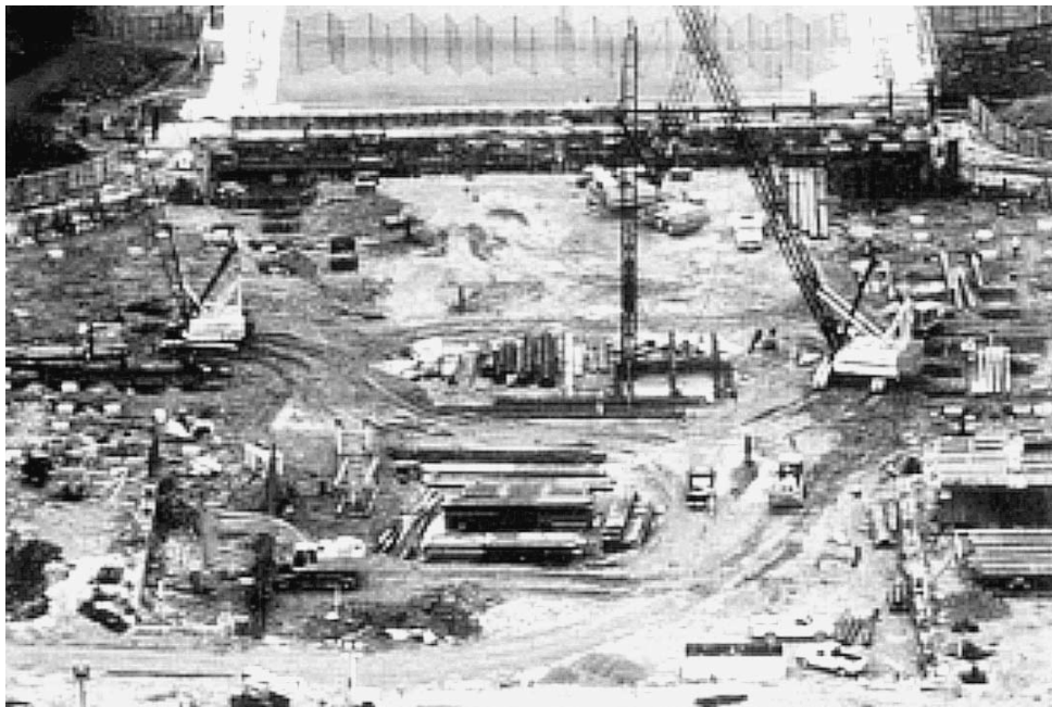
View of the National World War II Memorial construction site taken from the top of the Washington Monument. Completed white pile caps can be seen on the left and in the upper right.
