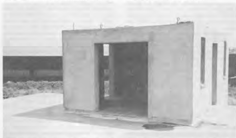
Top of Shipdham Tower which has been re-cemented and waterproofed. (Photo by Bert Carlberg, 67th Squadron)
